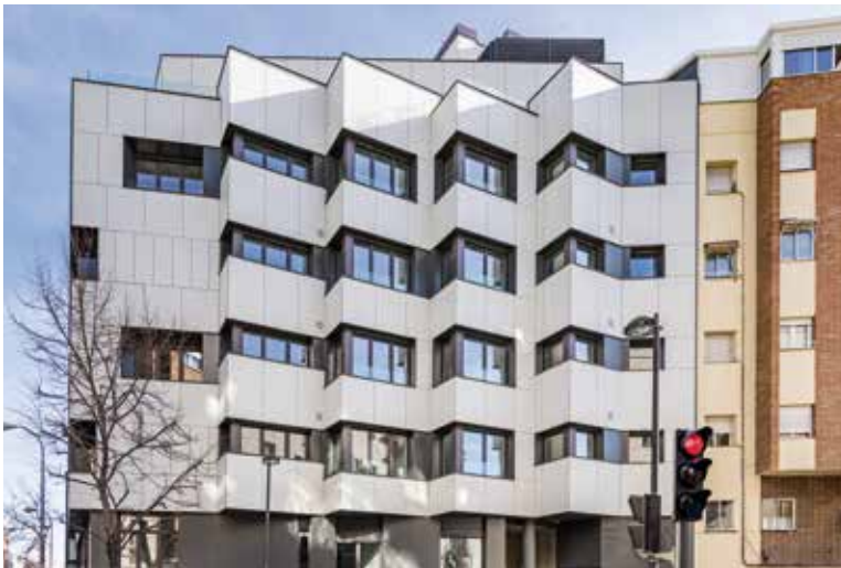
Photo: EnerPHit renovation standard achieved with 14cm of mineral wool in Madrid, Spain (residential building, Calle Cartagena, ID 6898)
