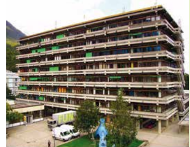
Photo: BEFORE renovation
