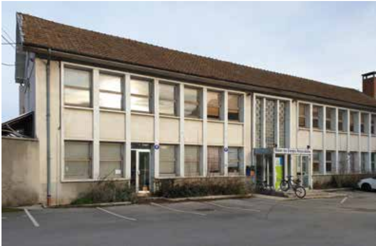
Photo: BEFORE renovation
