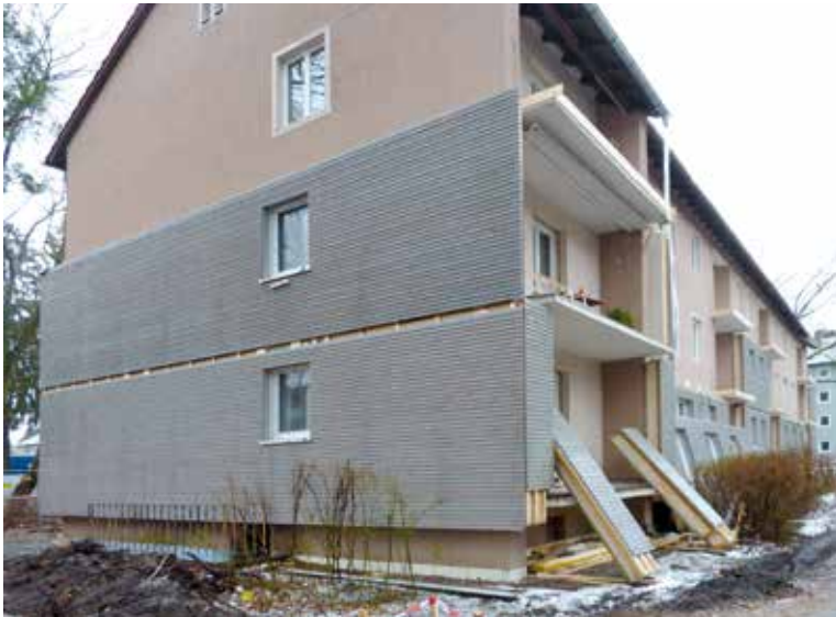
Photo left page, bottom right: Manually insulated loggias
