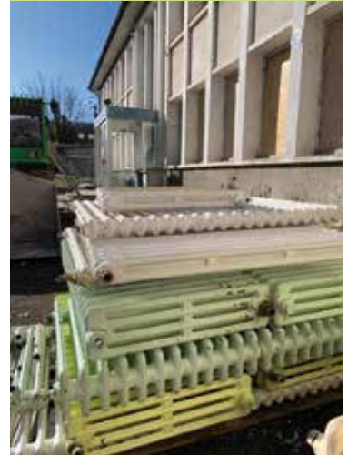
Photo above: The original radiators from 1960 were removed
