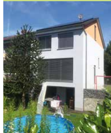
Photo: EnerPHit renovation in Laudens- bach, Germany (ID 4664)
