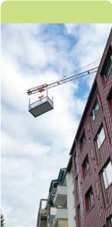
Photo above: Balconies mounted with a crane
