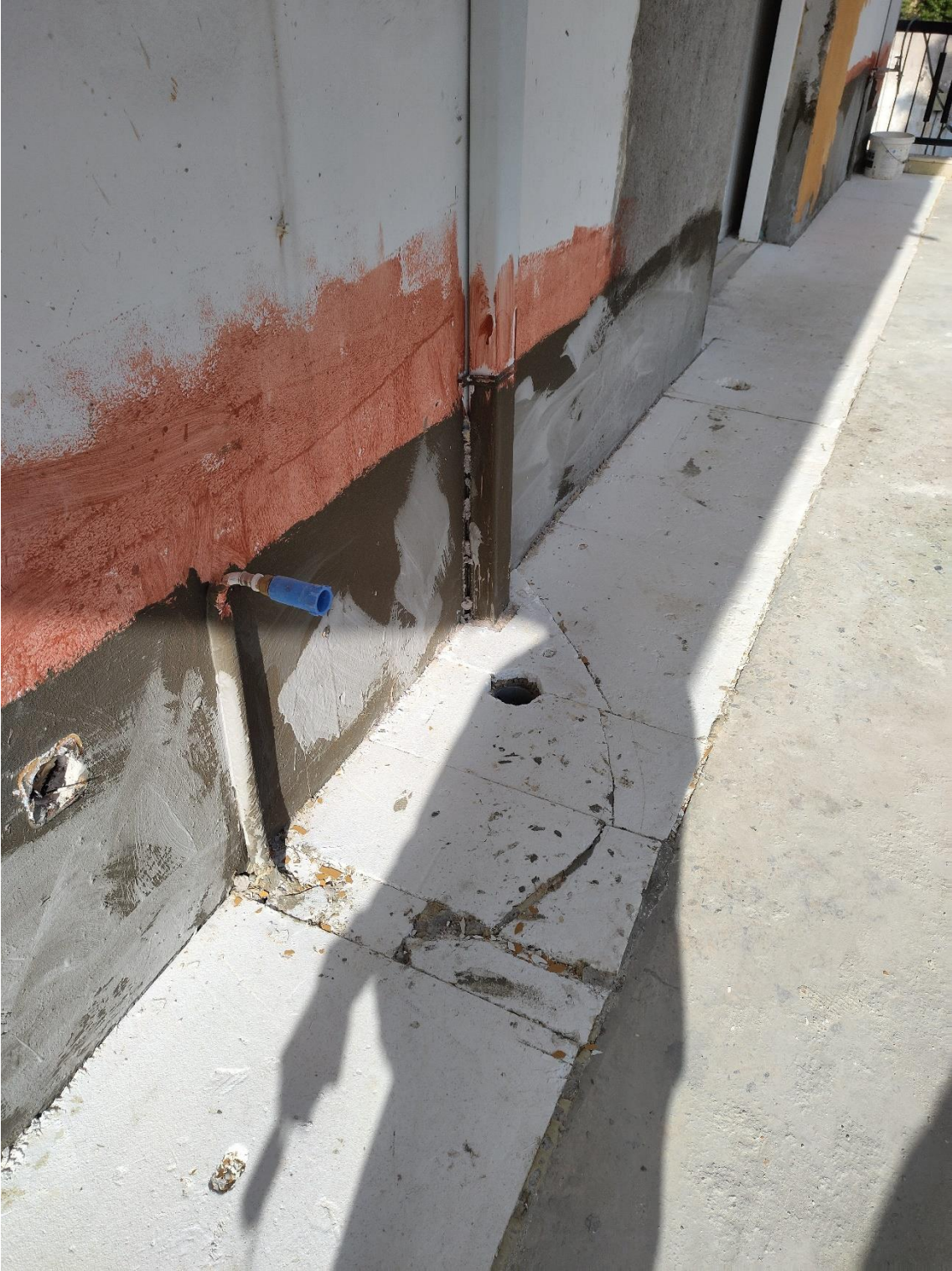
Figure 11 Installation of 60cm of insulation in order to minimize the thermal bridge in the balcony
