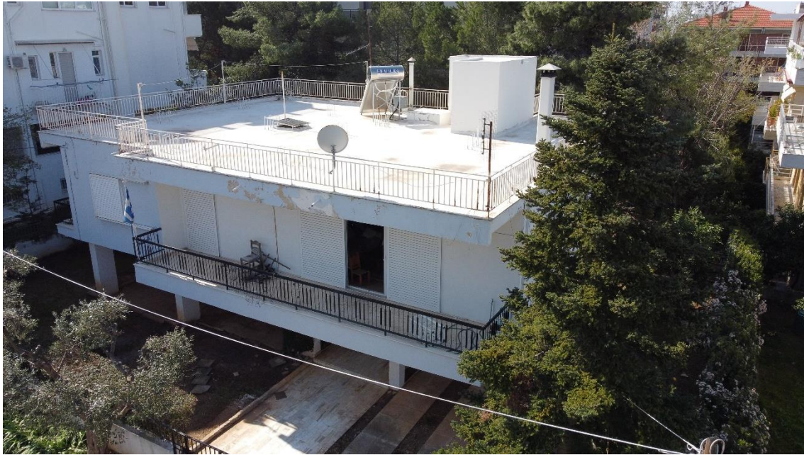
Figure 2 The existing building before the renovation
