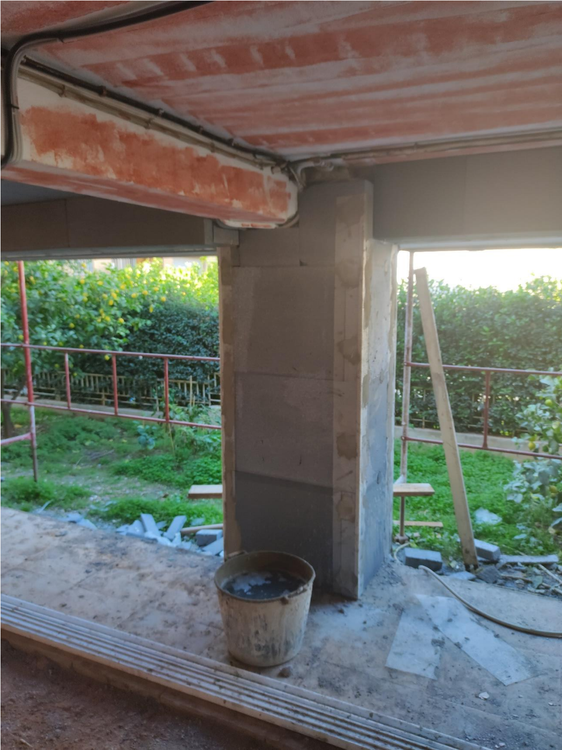
Figure 10 Eliminating the thermal bridges between the pillars and the pilotis
