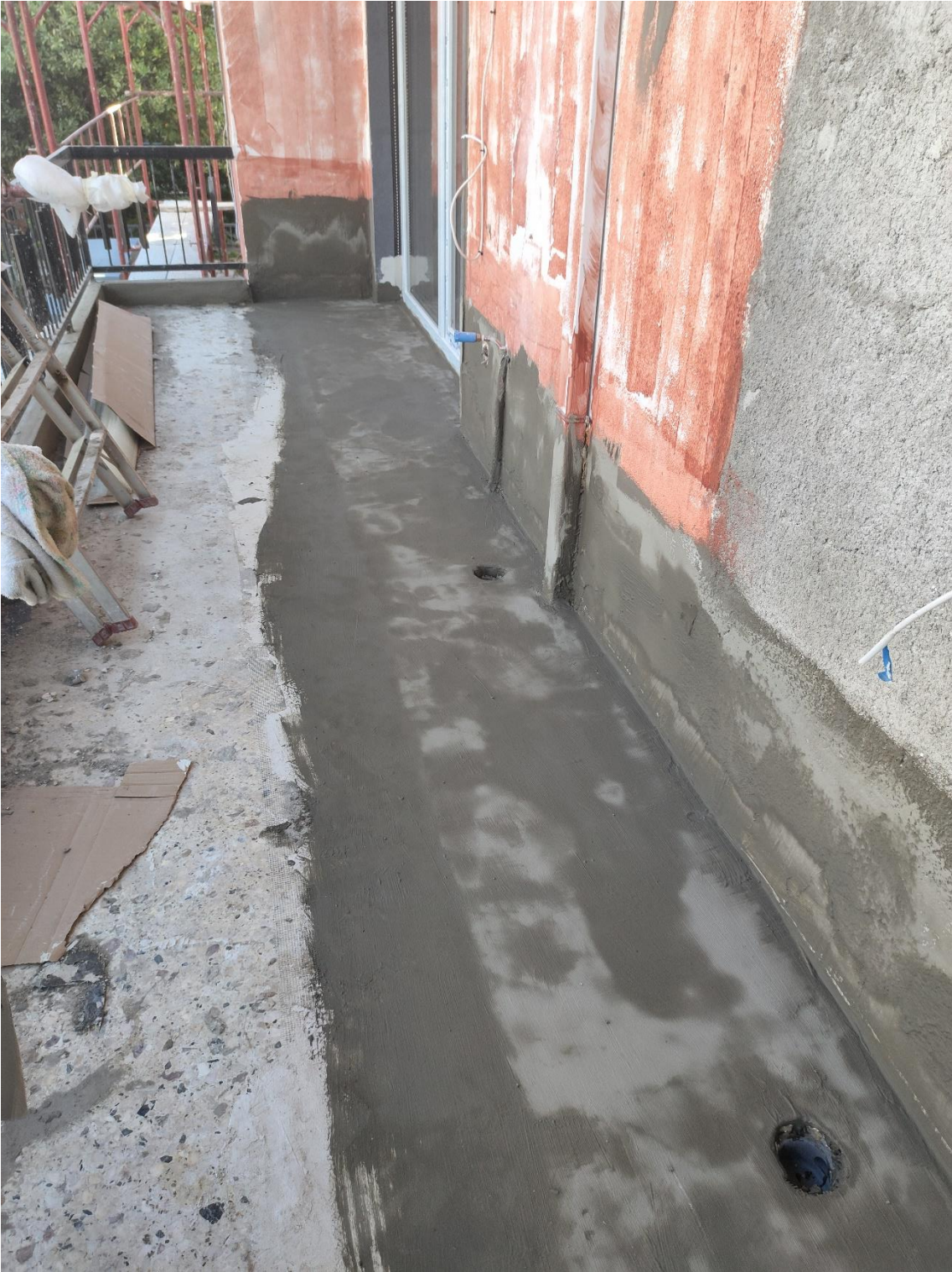
Figure 12 Installation of 60cm of insulation in order to minimize the thermal bridge in the balcony
