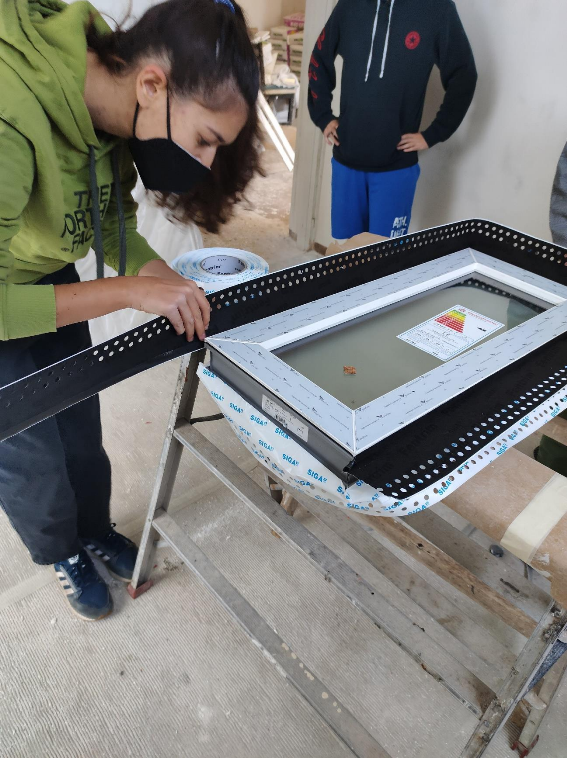
Figure 7 Installation of airtightness tapes
