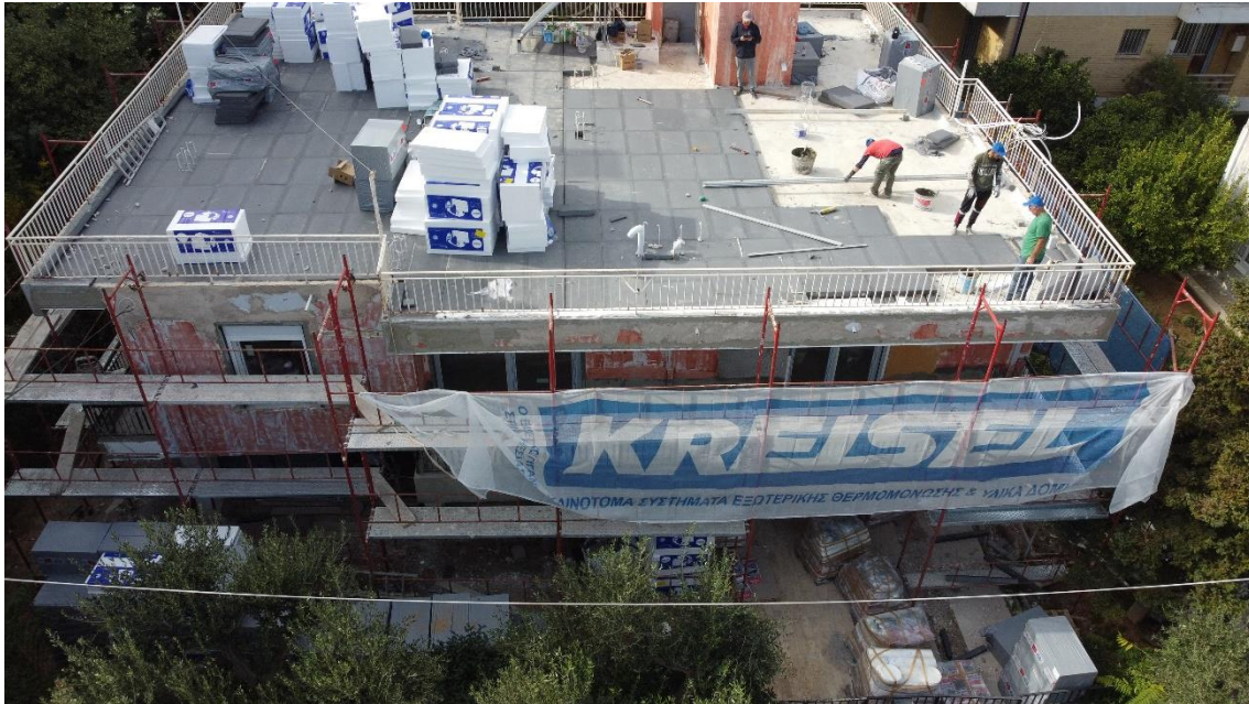
Figure 1 Photo taken during the installation of the roof insulation
