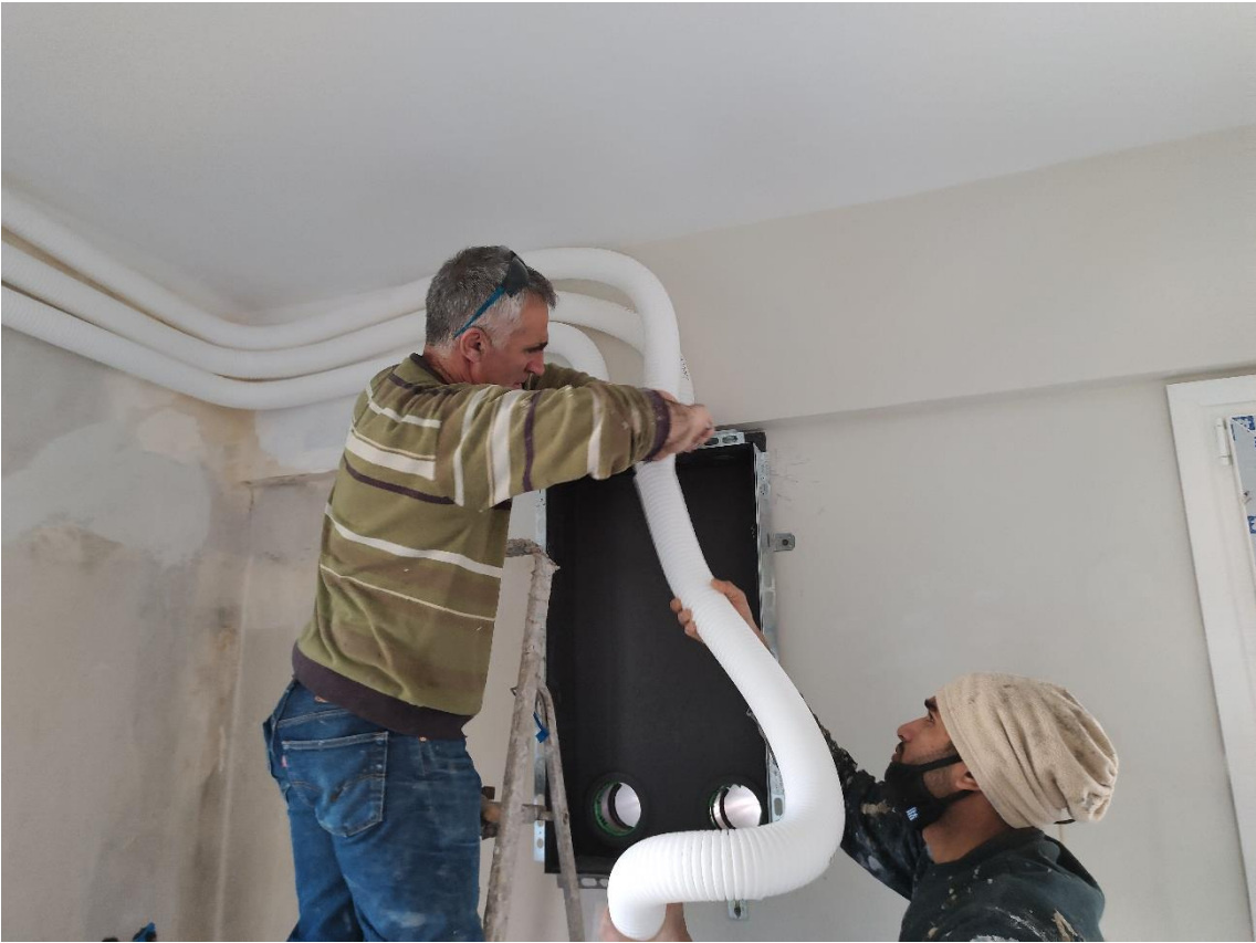
Figure 9 Installation of the MVHR and the air pipes
