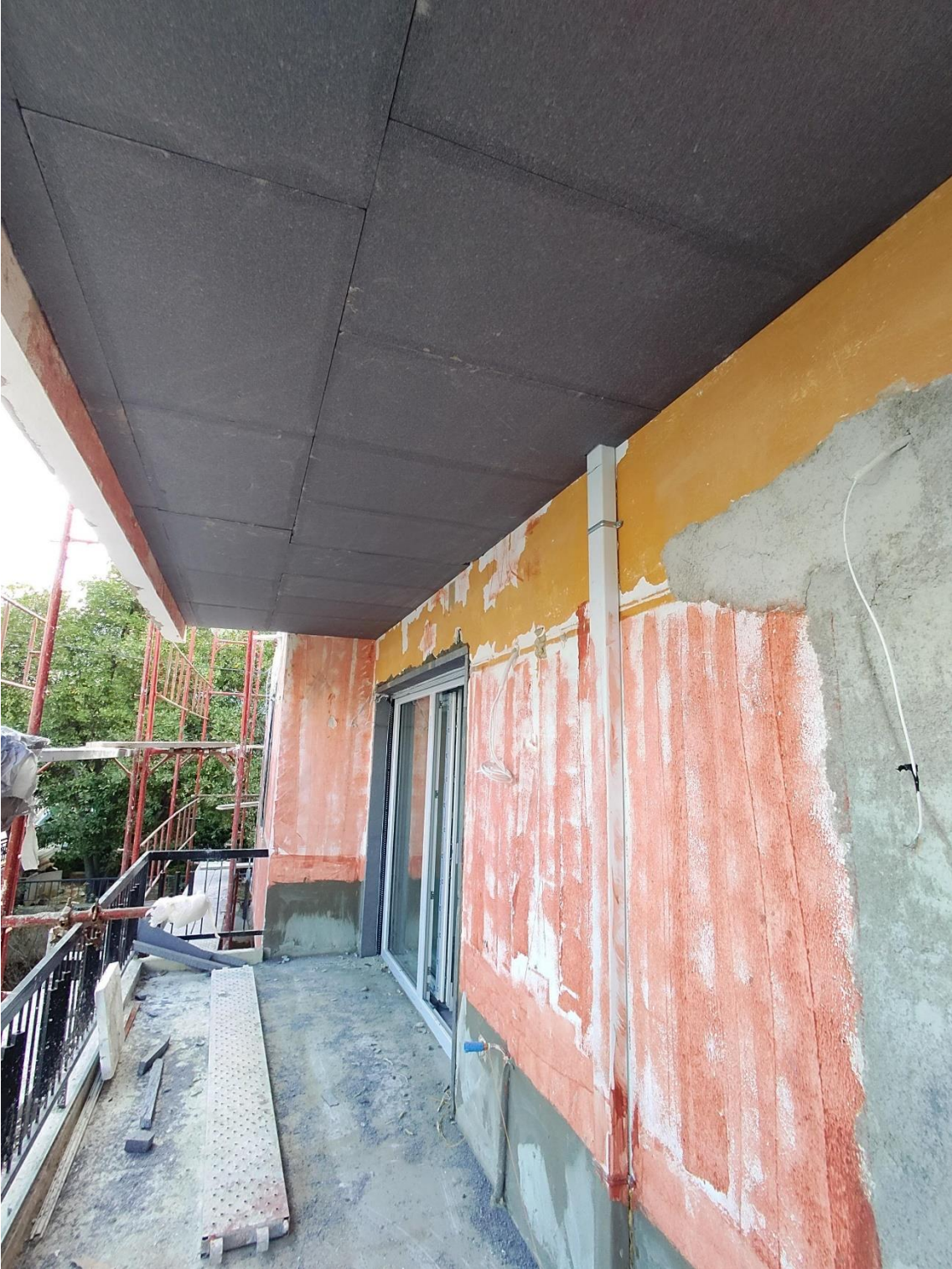
Figure 8 Installation of insulation in the down side of the extended roof
