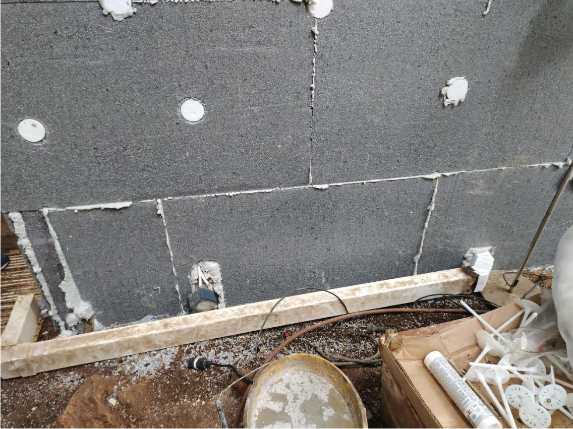
Figure 8 Installation of insulation
