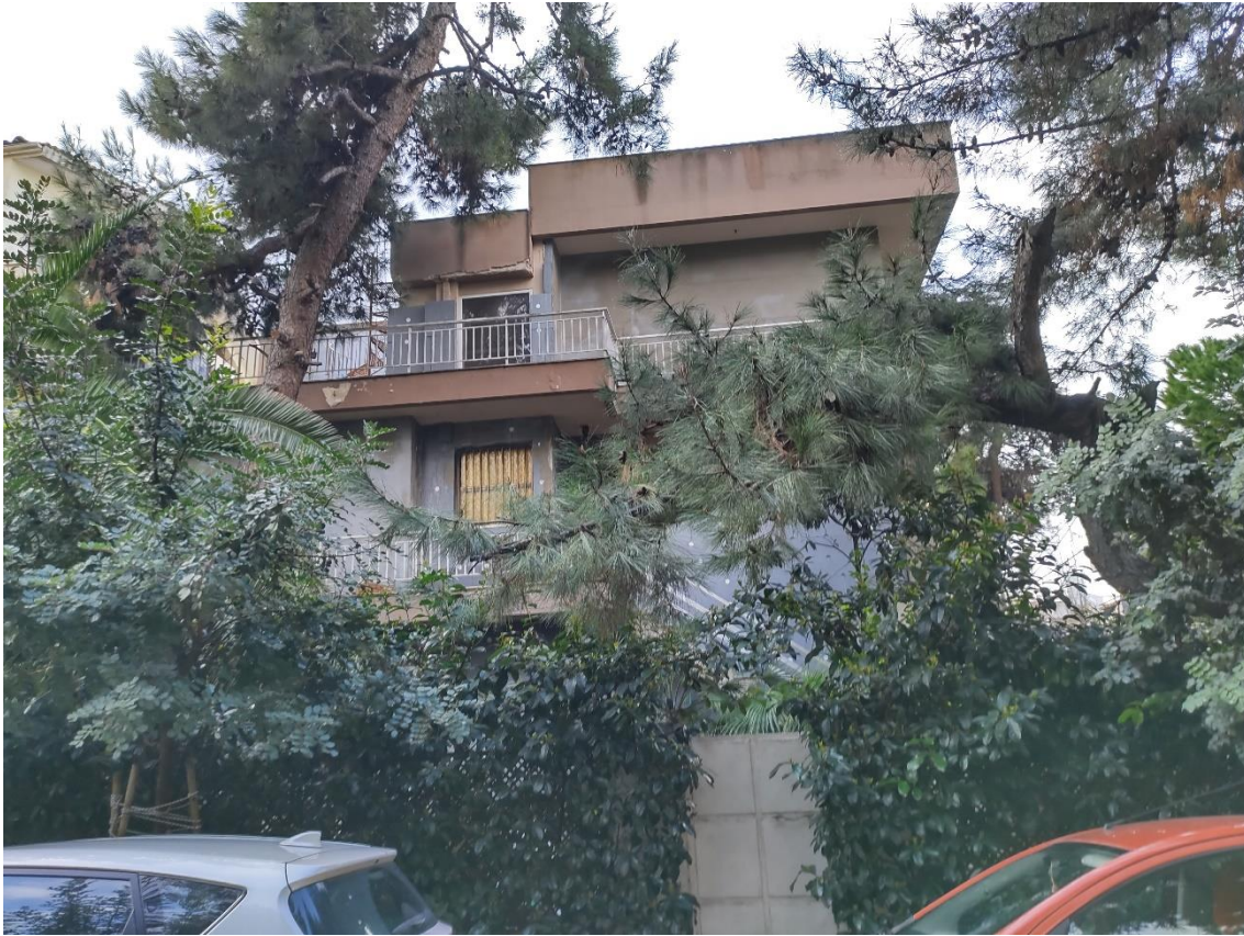
Figure 2 The existing building before the renovation
