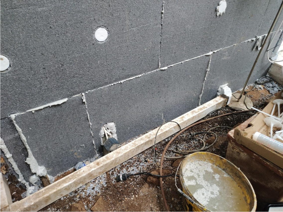
Figure 7 Installation of insulation
