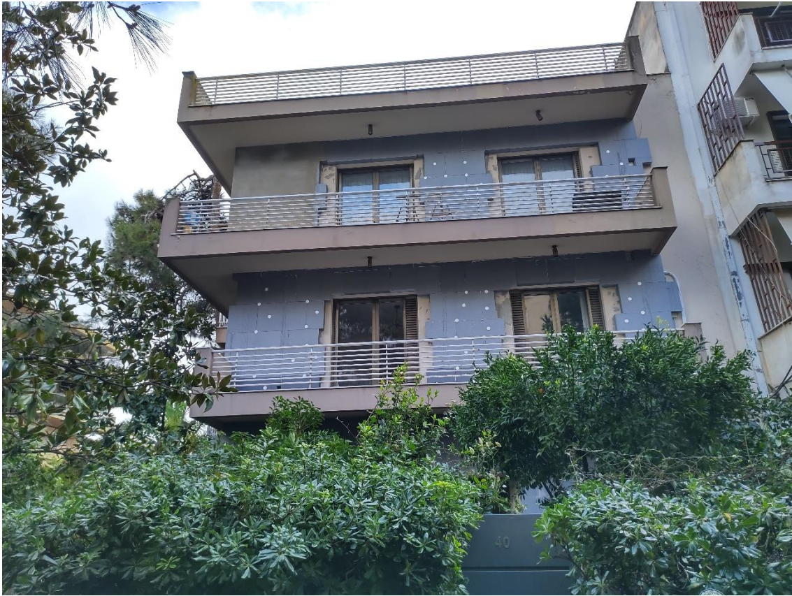
Figure 1 Photo taken during the installation of the wall insulation
