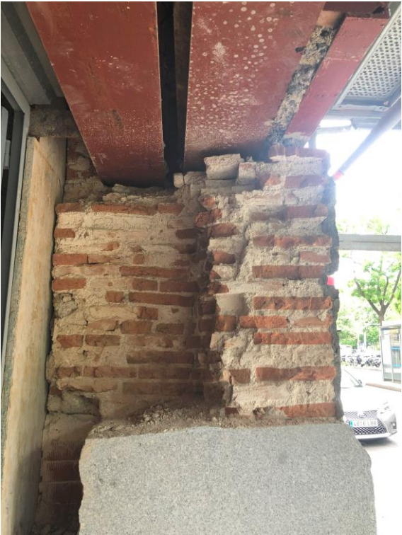
Protected historical façade @ VAND arquitectura
