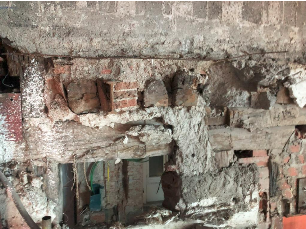
Exterior wall-interior ceiling connection. Existing situation @ VAND arquitectura
