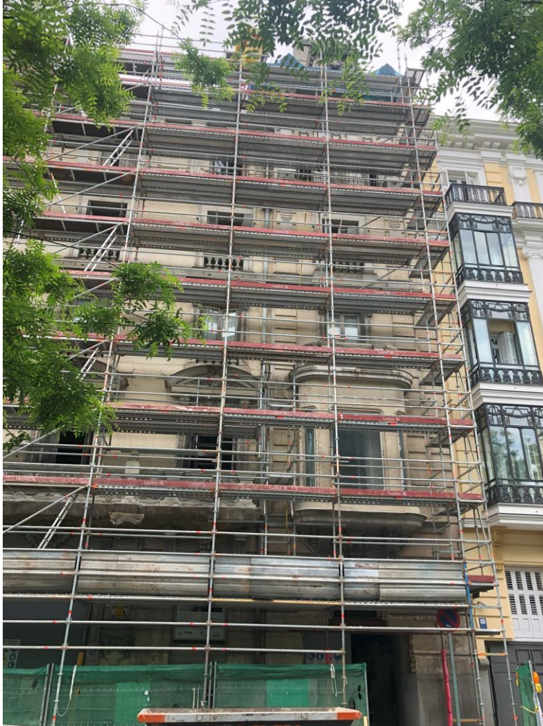
Protected historical façade @ VAND arquitectura
