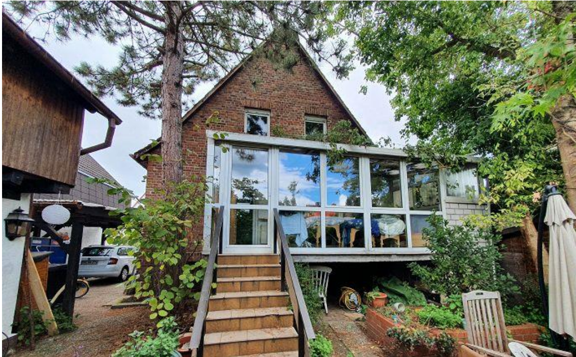
Back side with Wintergarden before renovation, Source: PHI
