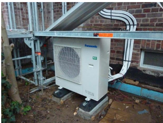
Heat pump and split unit during the installation, Source: PHI
