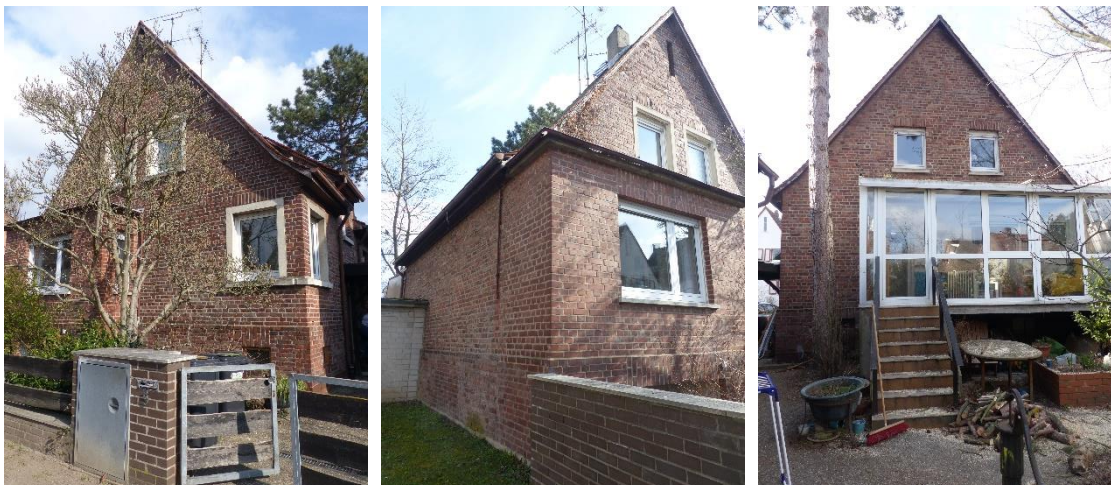
Existing Brick Wall Facade, Source: PHI
