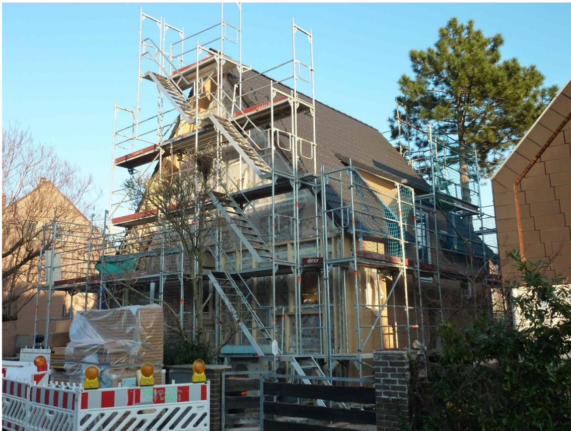
Street façade during the renovation of the building, Source: PHI
