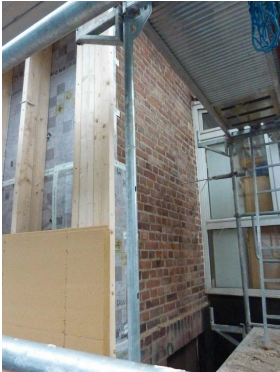
Old brick wall with stud wall system / Source: PHI
